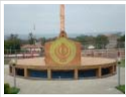
The detailed tiling work on the base of the new Nishan Sahib
